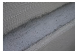
Filete redondo hecho de KÖSTER WP Repair Mortar
