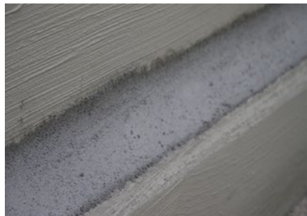
2 Media caña instalada con KÖSTER WP Mortar
