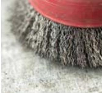
2 Prepare substrate by cleaning with wire brush and/or vacuum cleaning
