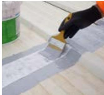
7 KÖSTER Superfleece can be embedded into the fresh layer on substrates that are at risk of cracking
