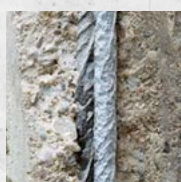
Corrosion protection (coating)
