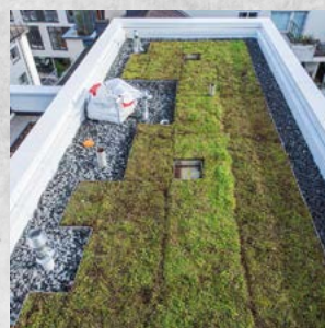
Under ballast / green roofs
