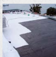
Waterproofing on bitumen
