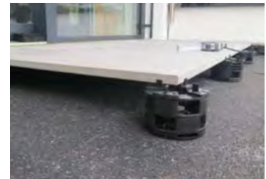
Tiles or paving on pedestal
