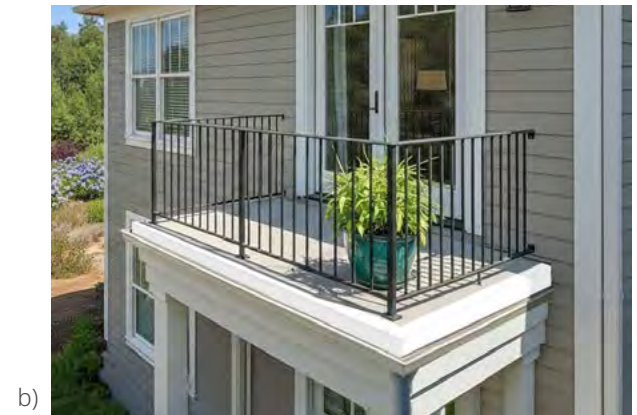
Balcony or terrace equipped with a drip edge and gutter to the drains
