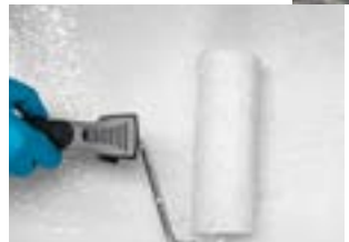
Apply it in two coats cross wise.
