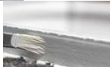
Apply it in two coats cross wise.
