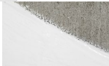
Apply it in two coats cross wise.
