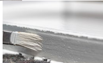
Apply it in two coats cross wise.
