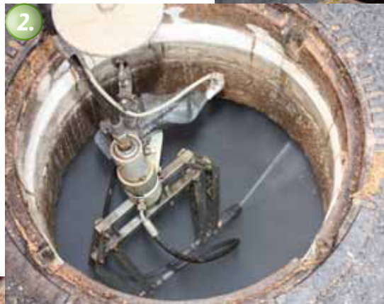
1. & 2. The substrate is prepare by high pressure water jetting (approx. 500 bar, depending on the site conditions)
