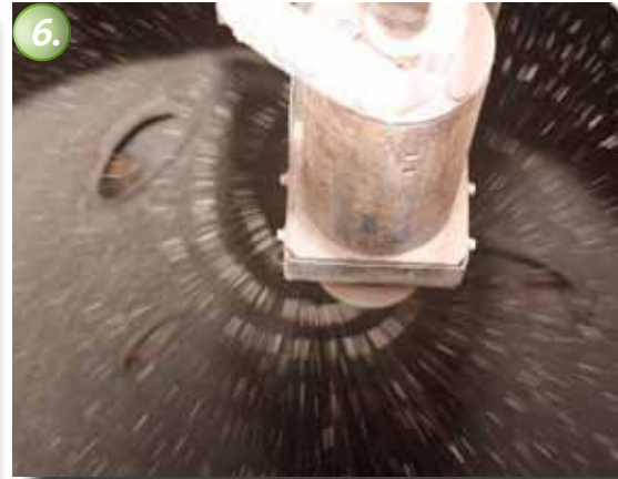
6. ...prepared substrate. this tool can be driven downwards and upwards in the shaft, therewith coating the shaft walls easily and very fast.
