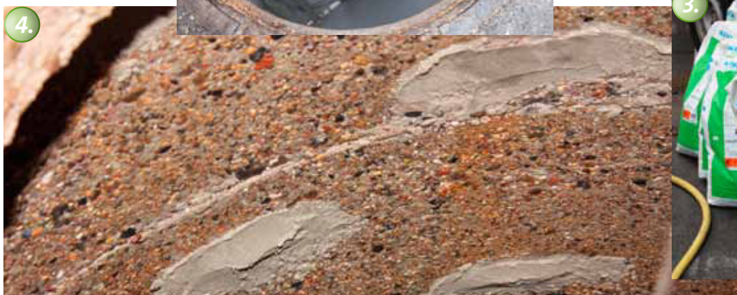
4. The substrate after water jetting. Break outs, voids are repaired. Old steel stairs have to be cleaned and treated with KÖSTER Z1 / Z2 Corrosion Protection.
