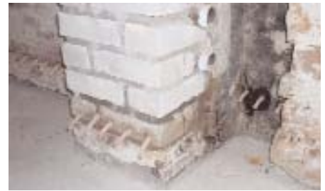
Fig. 8 a, b: Horizontal waterproofing at a listed building
