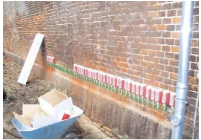
Fig. 8 a, b: Horizontal waterproofing at a listed building
