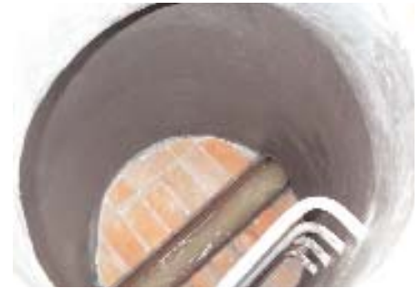
Fig. 10: completely renovated manhole after being coated with polymer silicate mortar (Photo: KÖSTER BAUCHEMIE)
